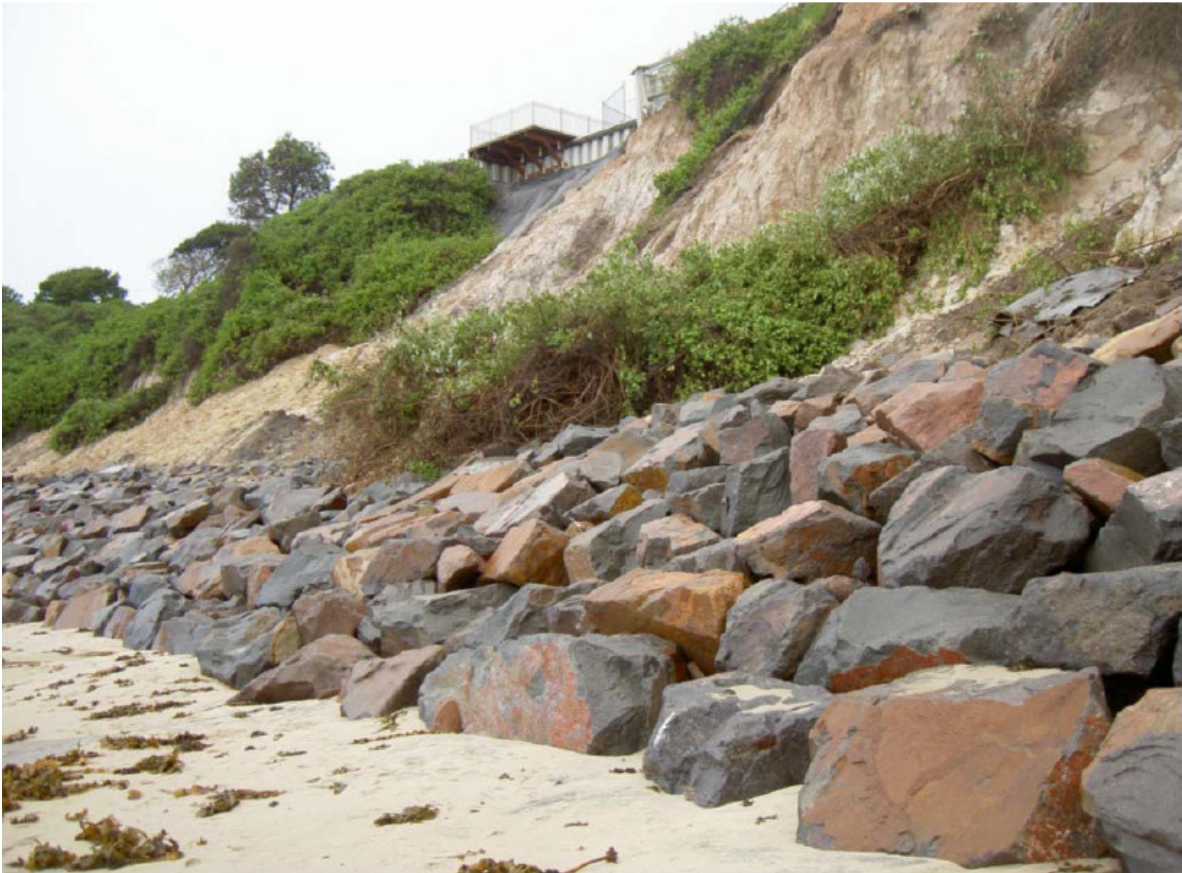
Figure 9: Completed Interim Structure at Cabbage Tree Bay, Norah Head, Wyong (Photo 2012 courtesy WorleyParsons)
